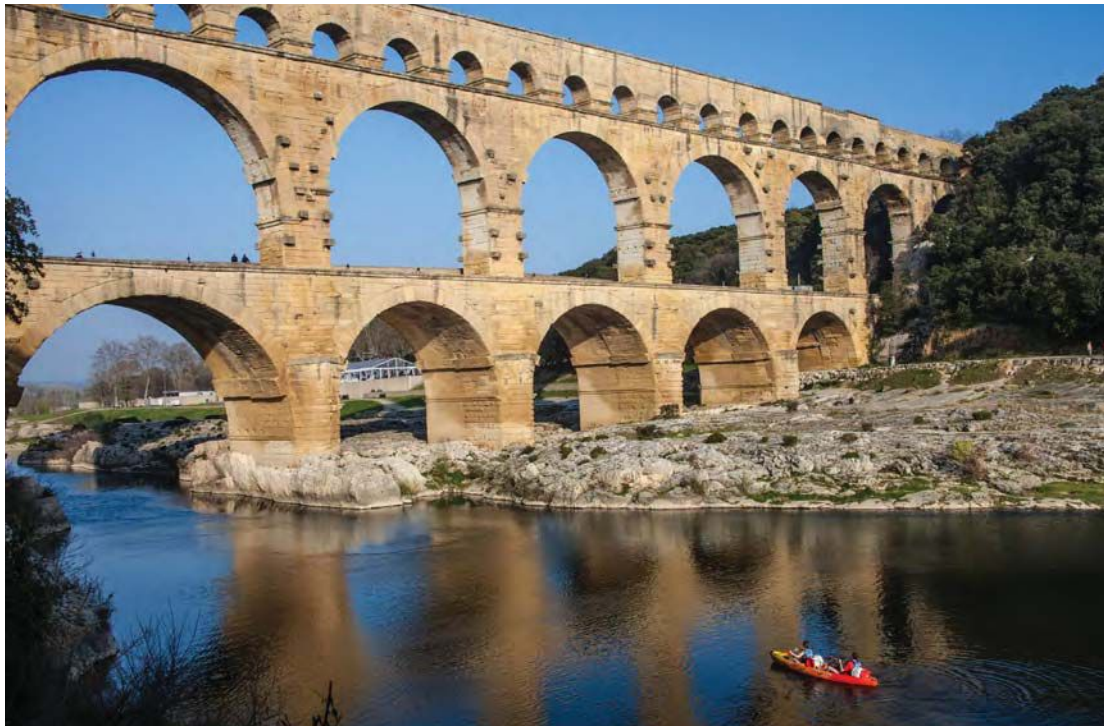
The Pont du Gard, a Roman aqueduct near Avignon, France, is a high point on Viking River Cruise tours.
